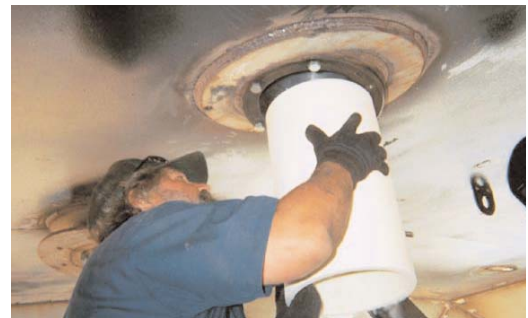
Installing SXL rudder bearing
